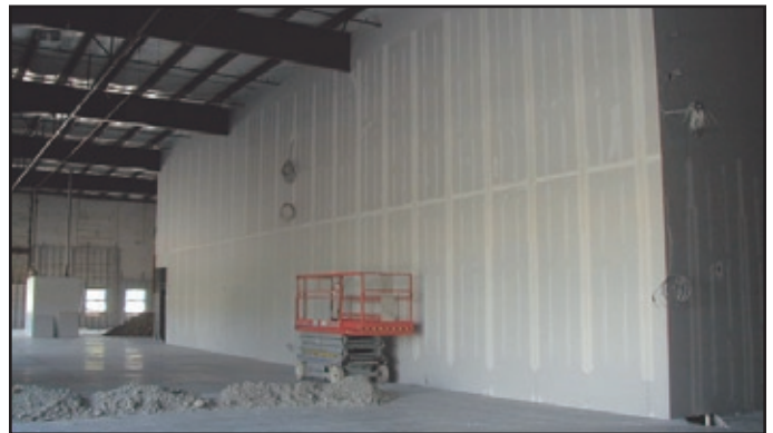
The walls are starting to go up!
