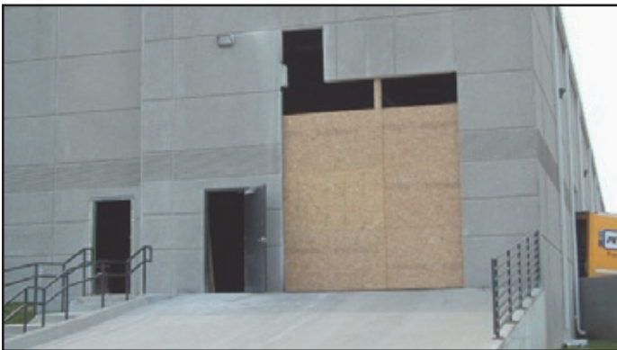
The training center will have a 22 ft. door.
